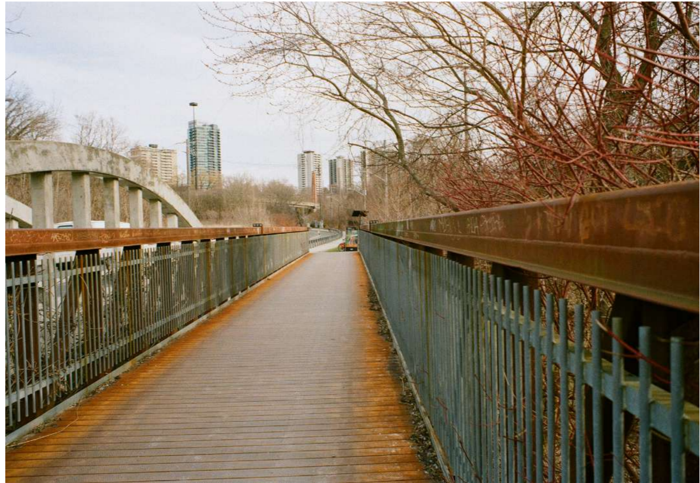
Pottery Road Bridge, April 2025
