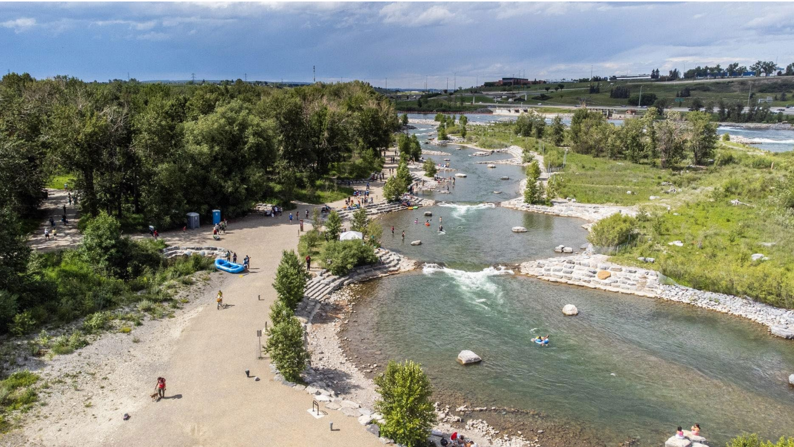
Photo: Harvie Passage Flood Damage and Repair, O2, CSLA Awards of Atlas
