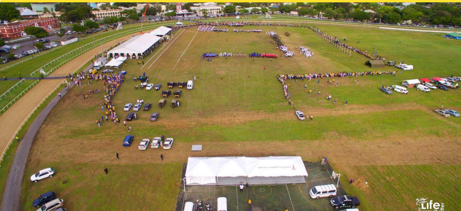
Fig. 11: Aerial View of Parade Square and hard court.
