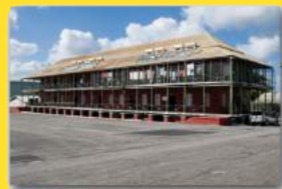
M243. Iron Barracks
